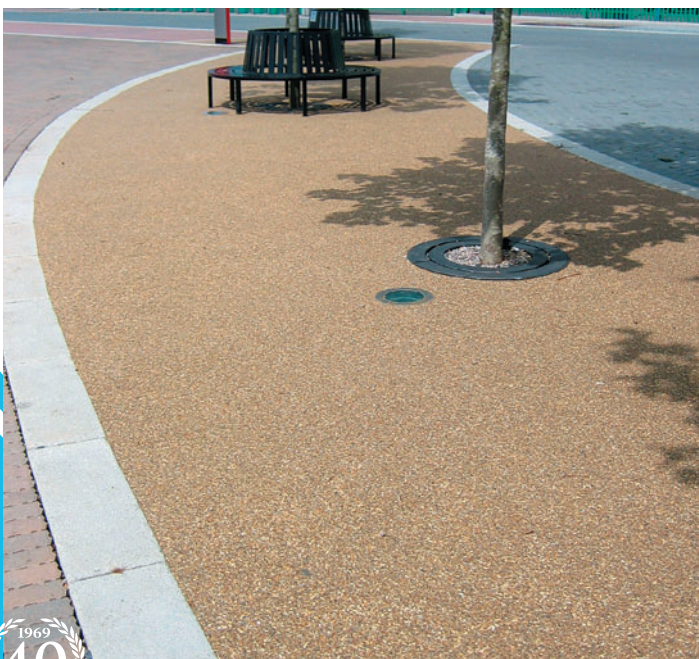
Resin bonded footpath and tree pit system
