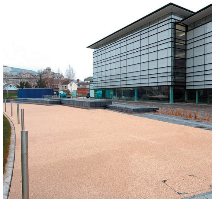
Resin bound pedestrian access road system
